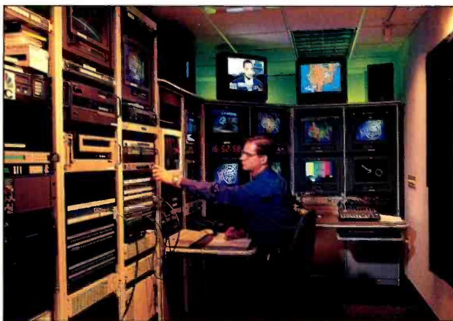
Master control for AccuWeather's WeatherTeam and WeatherTeam Live segments is equipped with a 16-input Grass Valley 1200 serial component digital production switcher.
