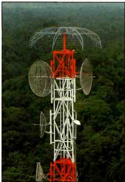
Lightning Eliminators and Consultants' Dissipation Array System, shown above, enables facilities to protect sensitive electronics from lightning strikes by utilizing the natural principle of charge transfer.
